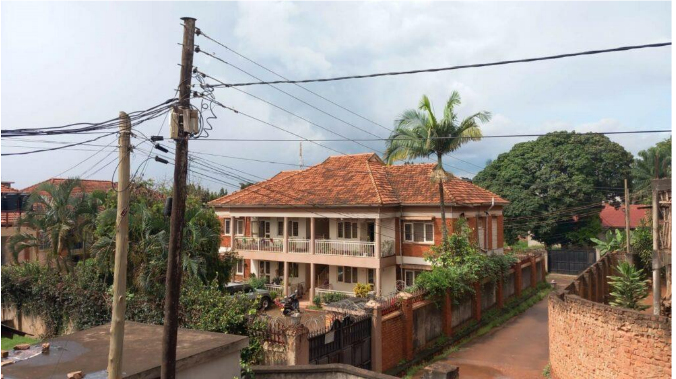
Electricity pole residential area in Kampala. Credits: Sarah Helen Rüdener.
