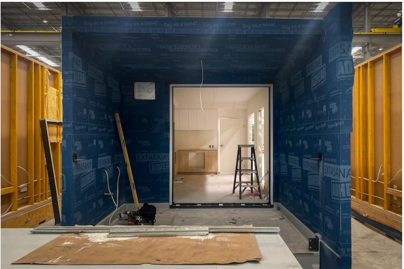
A prefabricated module for an apartment building bound for Queensland from a Melbourne factory. (ABC News: Rachel Clayton)
